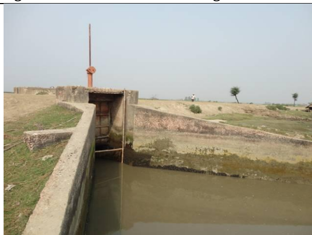
Figure 2: Betibunia 2vent Drainage sluice
