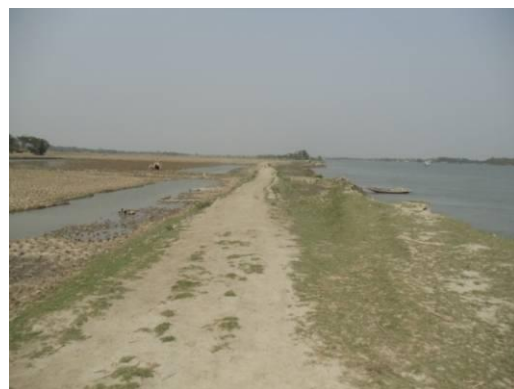
Figure 4.3: Daratana river bank erosion at Mollikerber
