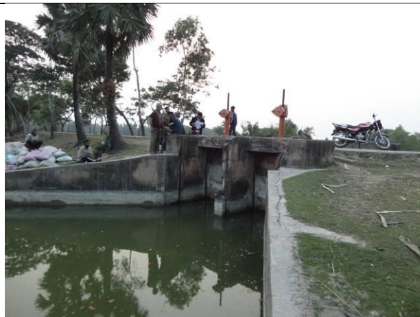
Figure 2: Betibunia 2vent Drainage sluice
