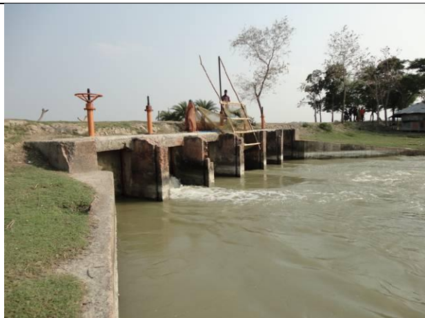
Figure1: Bashbari 6 vent Drainage sluice
