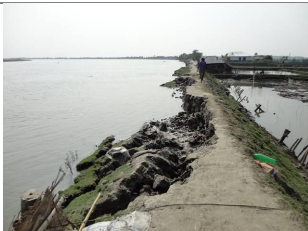
Figure7: River bank erosion at Radabhallob
