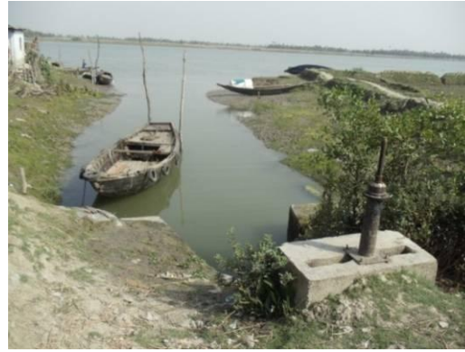
Figure 4.5: One vent sluice at Matherdia
