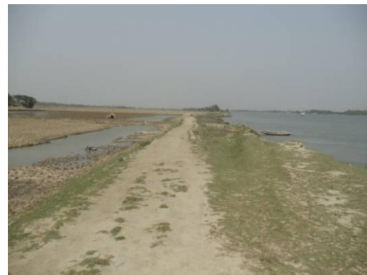
Figure 6.11: Embankment of the polder at Mollikerber
