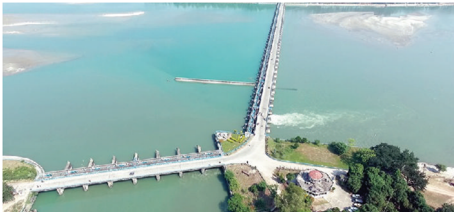
Teesta Barrage & Canal Head Regulator
